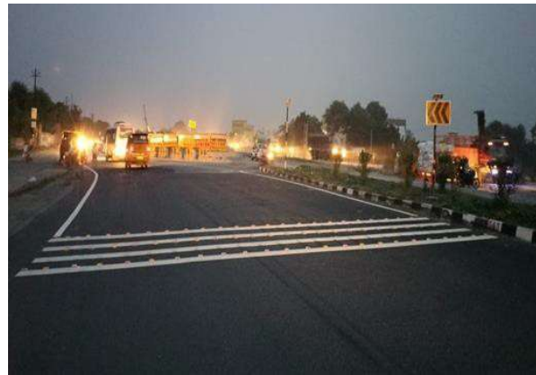
Road Diversion in the night
