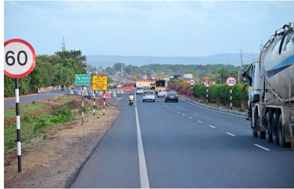
Road Diversion in Day Time
