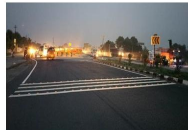
Road Diversion in the night
