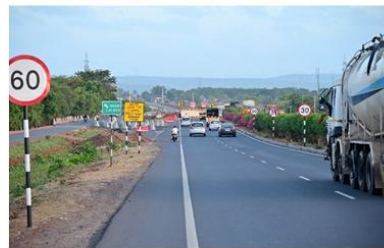
Road Diversion in Day Time
