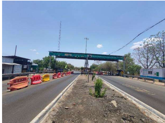
Kelapur Toll Plaza
