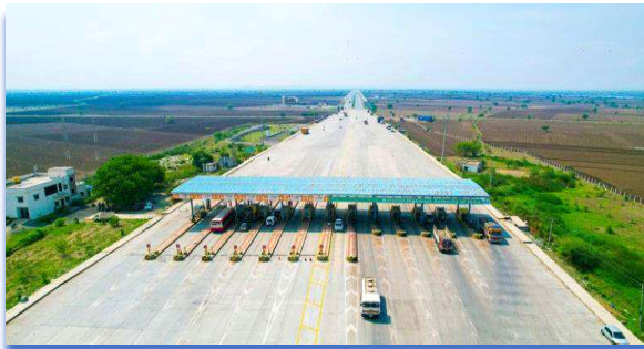
Bankapur Toll Plaza
