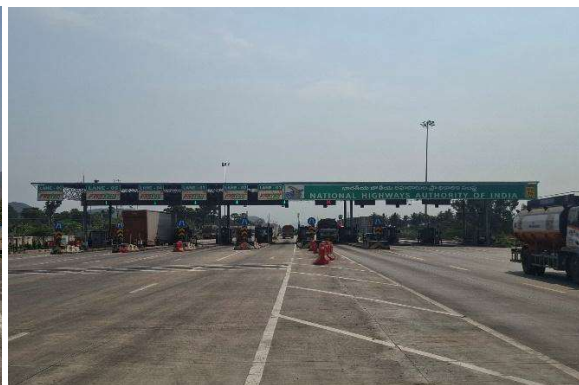
Marripalem Toll Plaza
