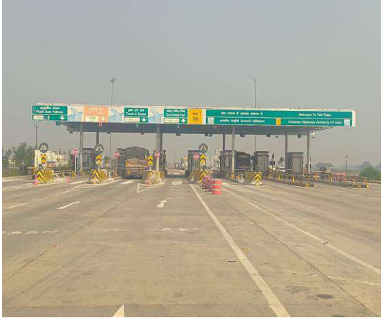
Odhaki Paipkhar Toll Plaza
