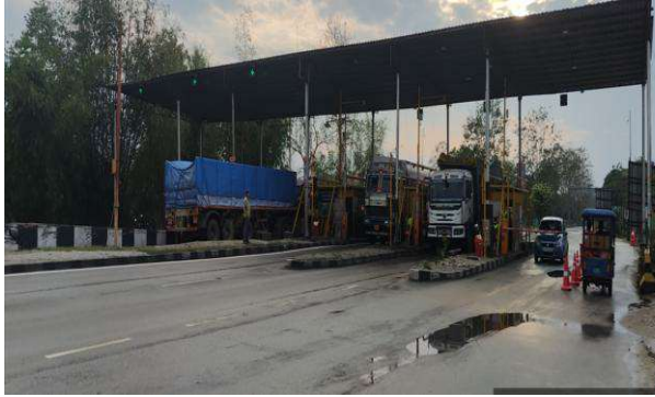
Patgaon Toll Plaza
