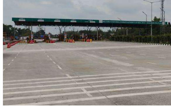
Dahalapara Toll Plaza
