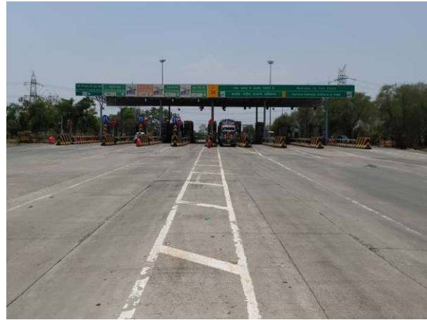
Boharipar Toll Plaza
