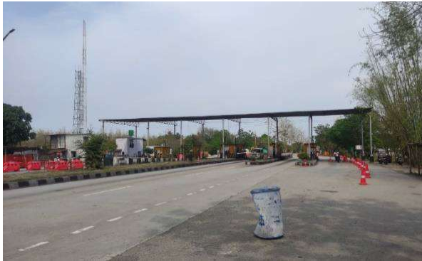
Patgaon Toll Plaza
