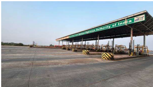
Bankapur Toll Plaza
