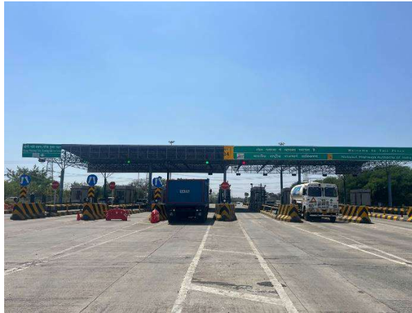
Boharipar Toll Plaza
