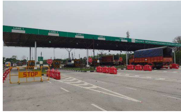
Dahalapara Toll Plaza
