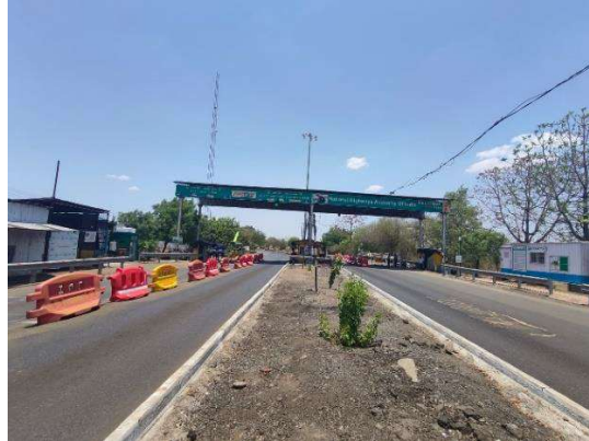
Kelapur Toll Plaza
