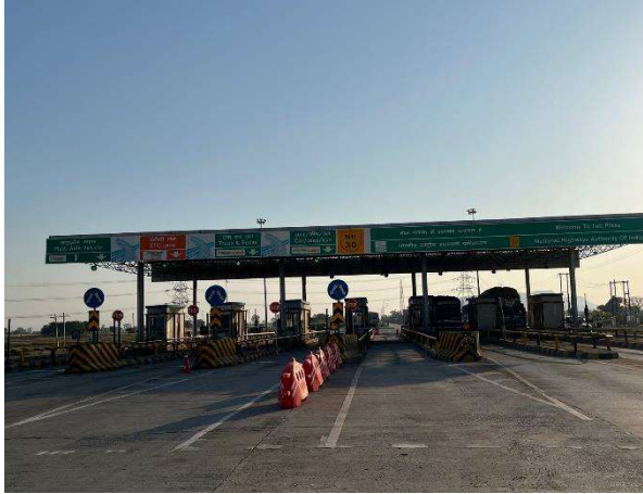
Odhaki Paipkhar Toll Plaza
