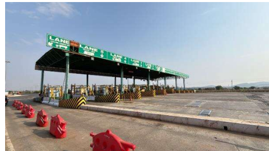
Chalageri Toll Plaza
