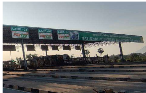
Marripalem Toll Plaza
