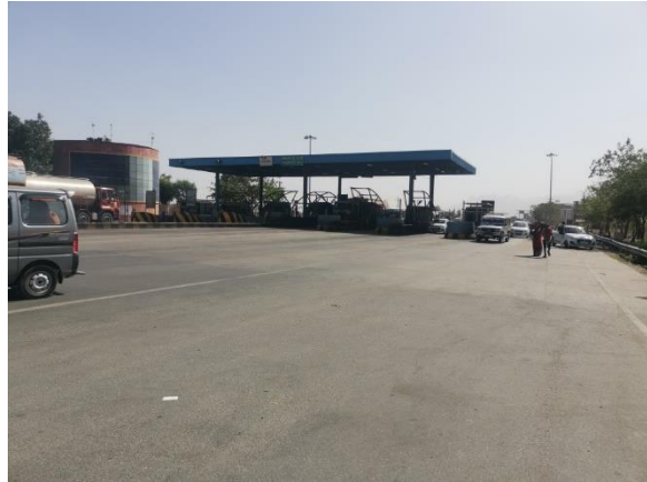
Undavariya Toll - Plaza
