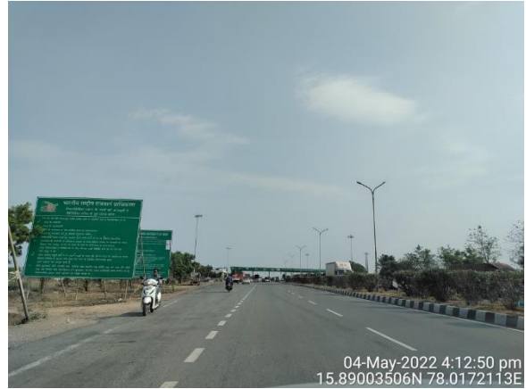
Pullur Toll Plaza
