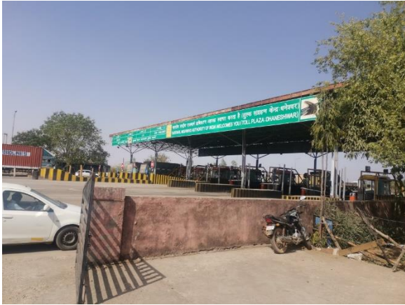
Dhaneshwar Toll Plaza
