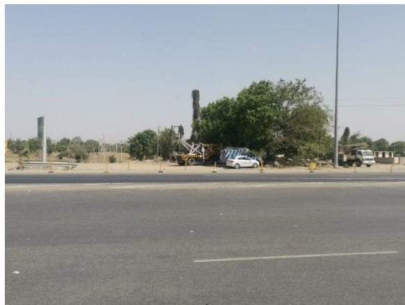
Palanpur to Abu Road Stretch
