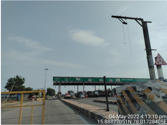
Pullur Toll Plaza
