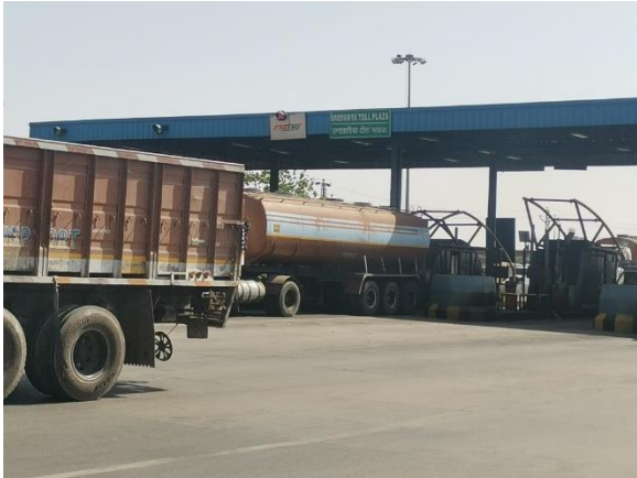
Undavariya Toll Plaza
