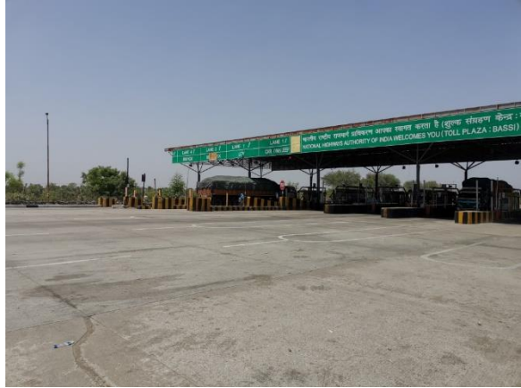
Bassi Toll Plaza
