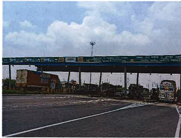
Raibha Toll Plaza
