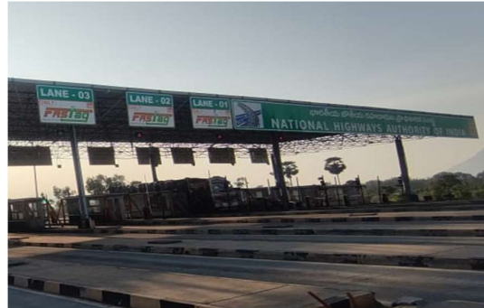
Marripalem Toll Plaza
