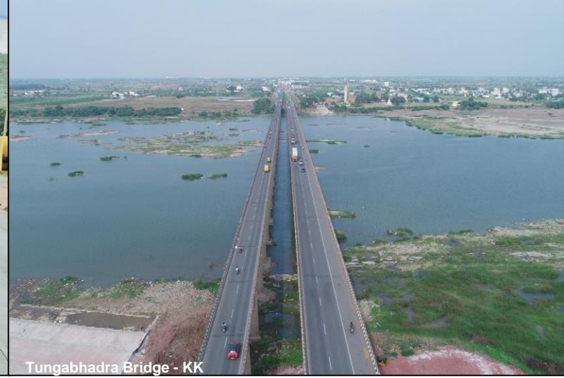
Tungabhadra Bridge - KK
