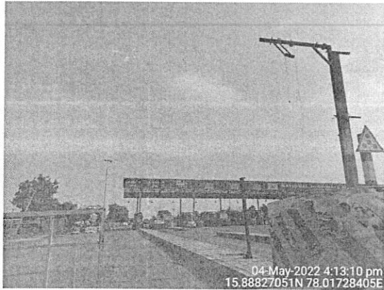
Pullur Toll Plaza
