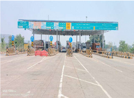
Kherwasani Toll Plaza
