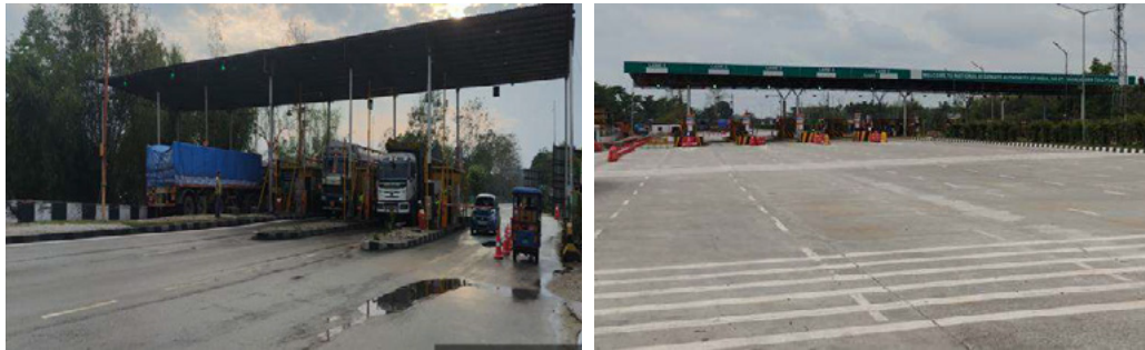
Patgaon Toll Plaza
