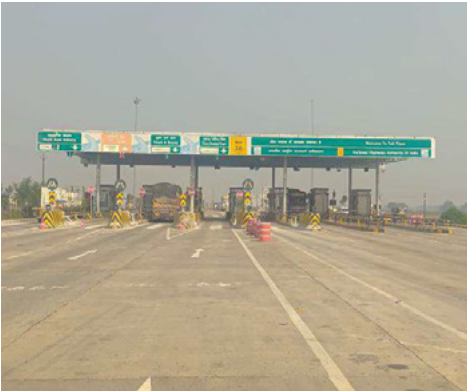
Odhaki Paipkhar Toll Plaza
