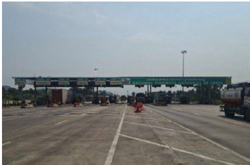
Marripalem Toll Plaza
